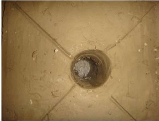
c): Pouring of crush stone
