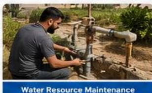
Water Resource Maintenance
